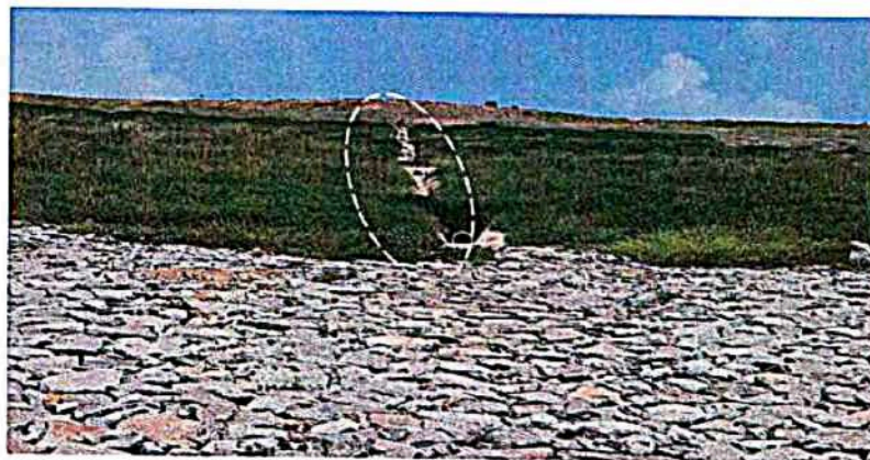
Figure 6: Cross drains on downstream slope at Ch. 13.6 km
