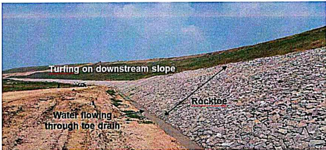
Figure 2: Downstream toe of dam at Ch 13.0 km.
