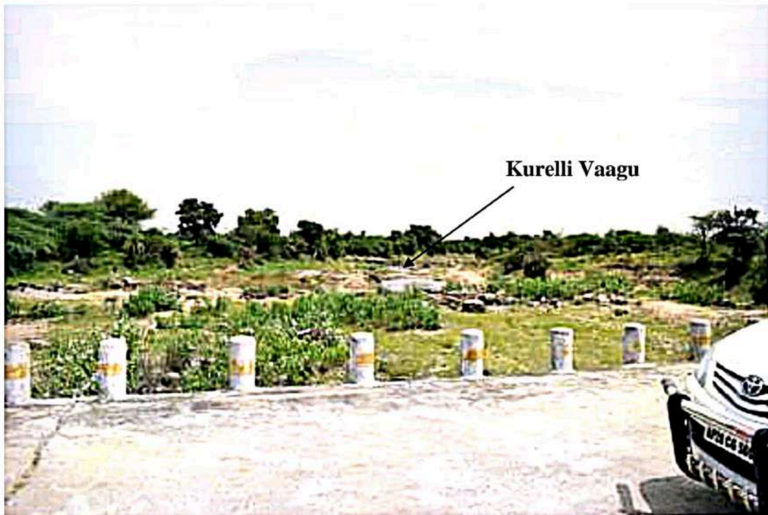
Photo 3: Existing bridge on Kurelli Vaagu stream.
