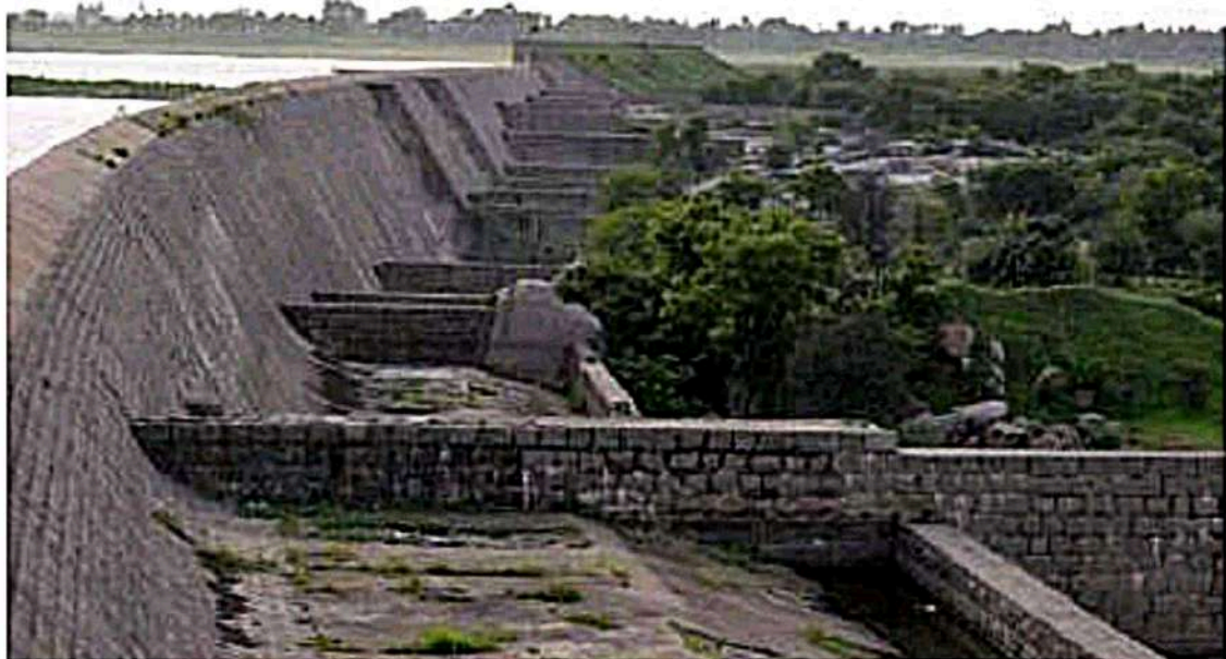
Photo 5: View of existing dam of Upper Maner reservoir
