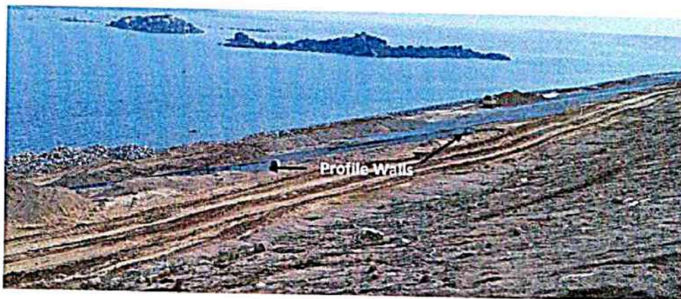
Figure 8: Upstream slope of earth dam at Ch. 15.6 km
