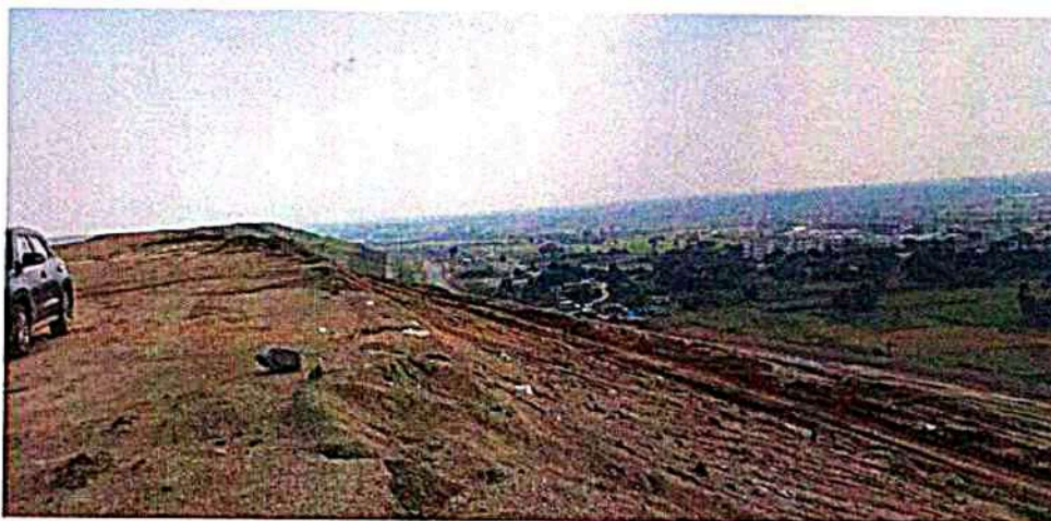
Figure 9: Downstream slope of earth dam at Ch. 15.6 km
